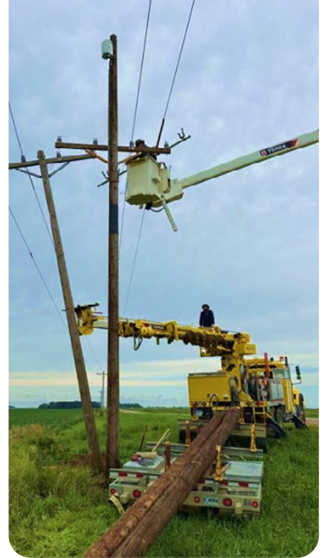
MINNEOTA – INSTALLING METER COLLECTORS OR REPEATERS
