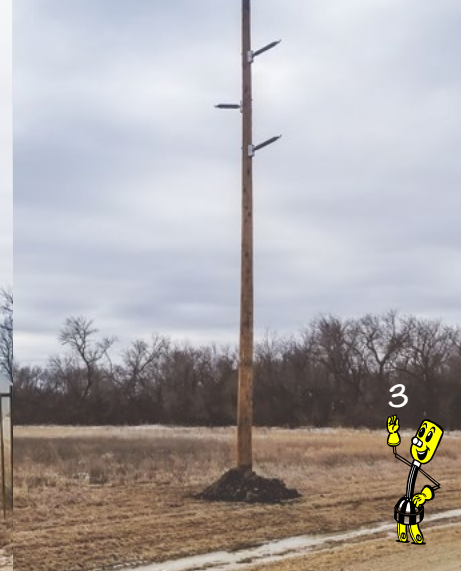
These are the first poles of the five mile project.
