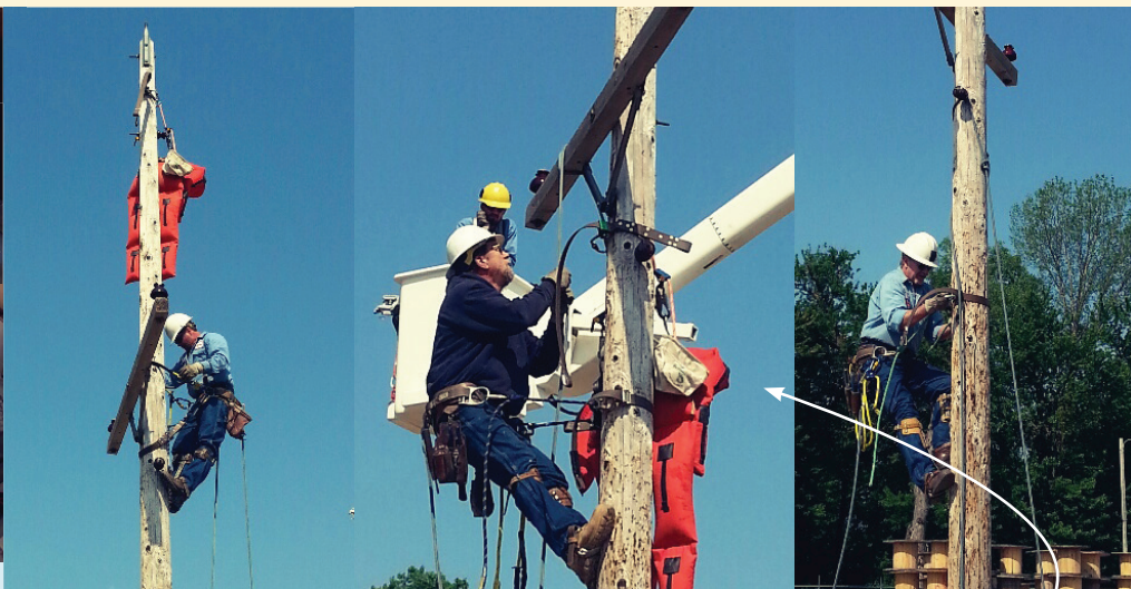
This past month, we held our annual pole top/bucket rescue proficiency testing. Kent Smith, Loyd Canatsey and Joe Schultz are pictured here rescuing a dummy.
